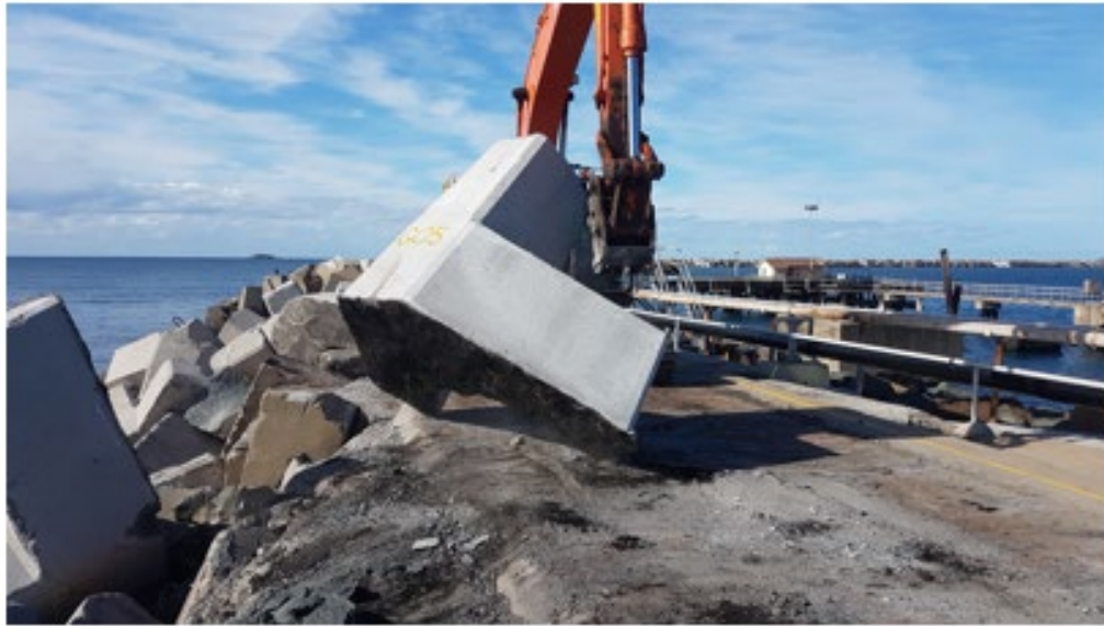
High Density Breakwater Armour Units
