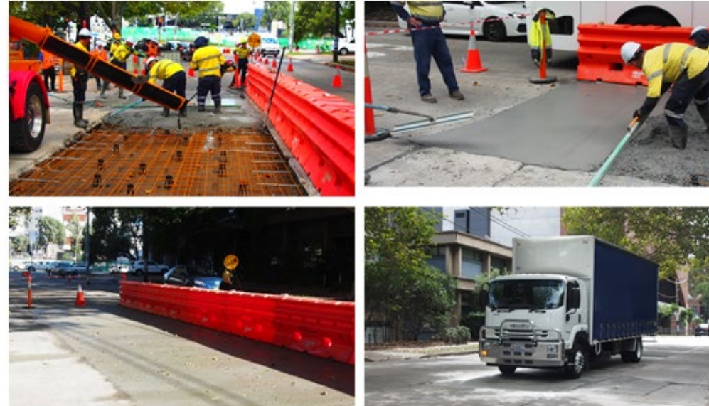
City of Sydney Pavement Trial
